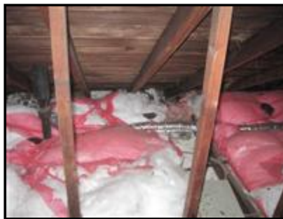
F. Picture 1 Insulation in soffit vents
